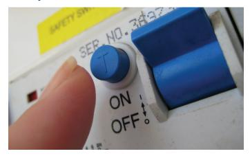
Have an electrician install safety switches on every circuit in your home. Don't mistake circuit breakers for safety switches. Circuit breakers are designed to protect circuit wiring and equipment, while safety switches protect people. A safety switch can be identified by its test button. If you can't see any test buttons, call your electrician. Remember to test your safety switches using this button at least every three months.
