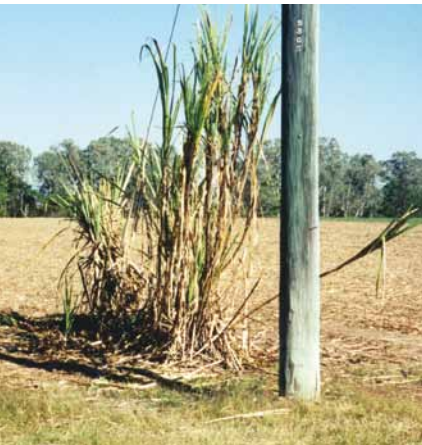
Keep all crops and vegetation well clear of power poles and stay wires.
